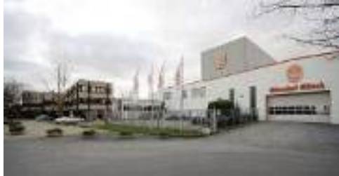
Image 1: Private brewery Reissdorf is re-located in Rodenkirchen in 1998. In 2008, Westfalia enlarged the capacities of the distribution warehouse for Kölsch in bottles and barrels more than 30%.
